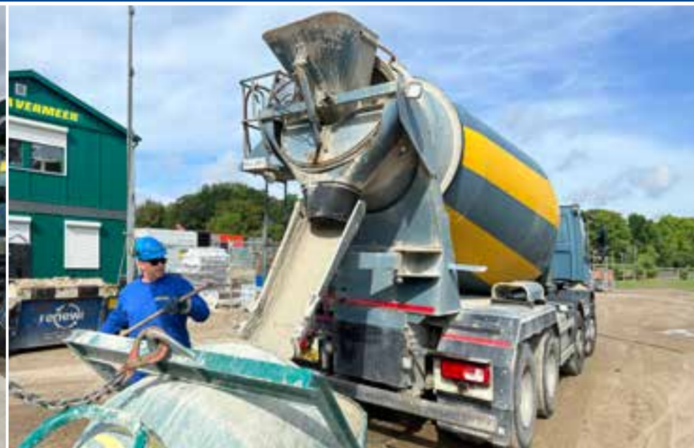
Albeton in werking
