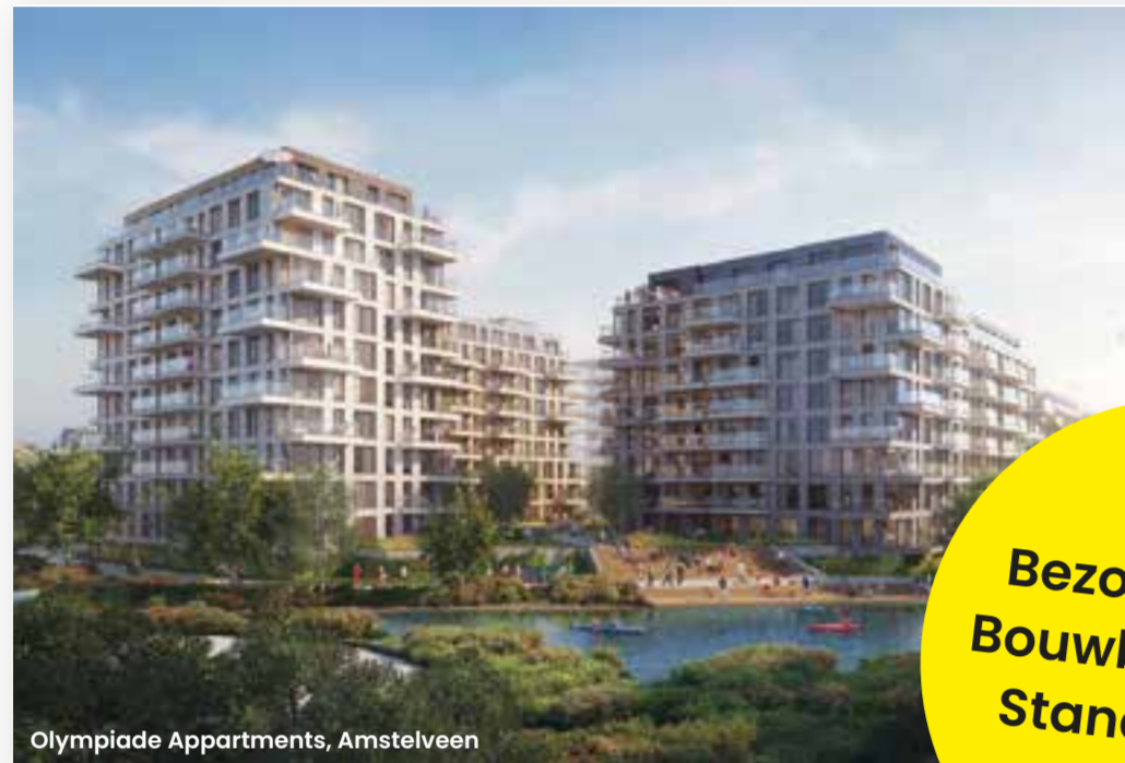
Olympiade Apartments, Amstelveen
